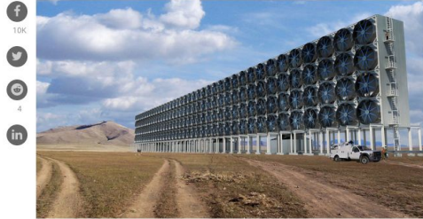
Banks of fans blow air through a carbon dioxide-capturing solution in this rendering of a direct air capture plant. CARBON ENGINEERING
