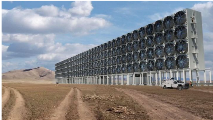
A rendering of Carbon Engineering's 'air contactor' design. The company uses carbon-capture technology that captures CO 2 directly from the atmosphere, and synthesizes it into clean transportation fuels. (Carbon Engineering)
